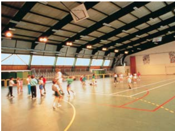
EZF is used both for total and spot heating in this sports centre. The hall is divided into different temperature zones to meet different temperature demands.
